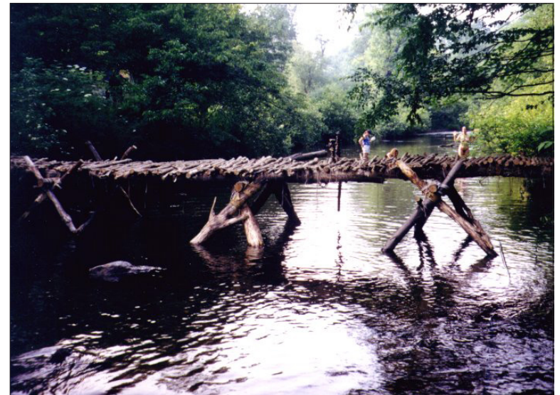
Homemade bridge, Pennsylvania 1999. Photo by Rob Savoye.
