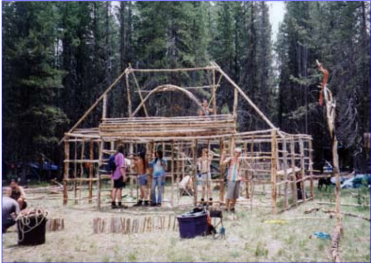
Granola Funk Theater under construction, Idaho 2001. Photo by Rob Savoye.
